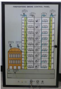
The FSCS is a manual control panel used for monitoring and overriding all smoke control equipment in a building. It provides firefighters with information about the state of the smoke control system as well as manual control over all of its components. The panel consists of command switches and LEDs as well as a custom diagram of the building that clearly indicates the type and location of smoke control equipment.
